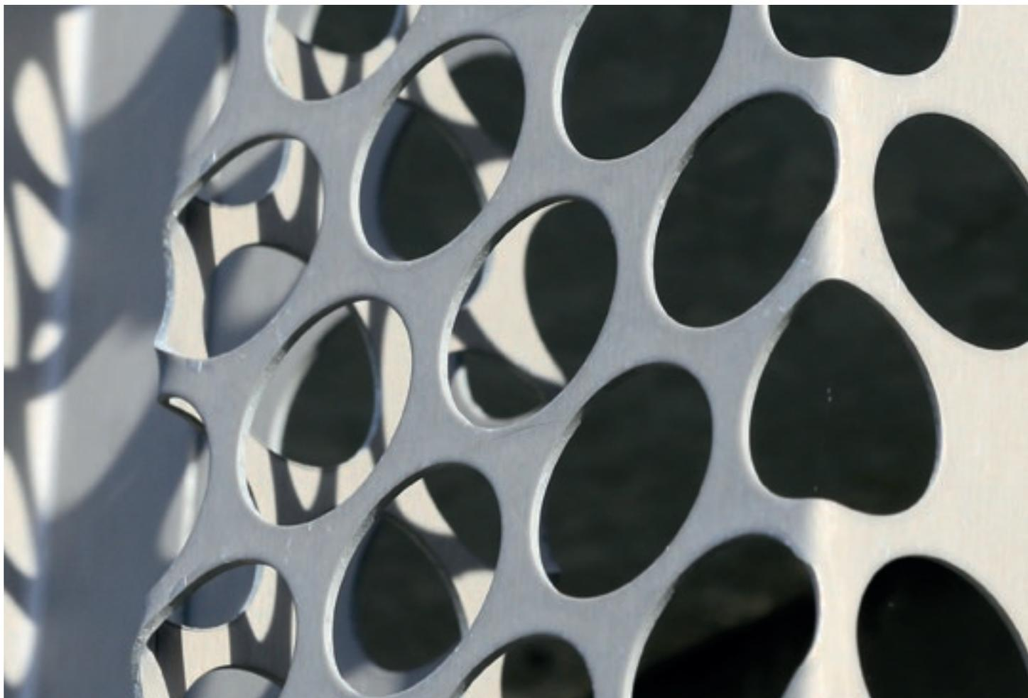
Thanks to its self-protective properties, perforated zinc acquires a natural patina. There is no risk of corrosion on cut edges. The intrinsic qualities of zinc make it an ideal material for perforated cladding systems. The elegance and lifespan of the project are ensured over the long term.
